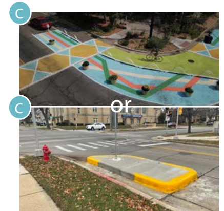
C. Interim Curb Extensions i. Paint-and-Post ii. Pin-on concrete
